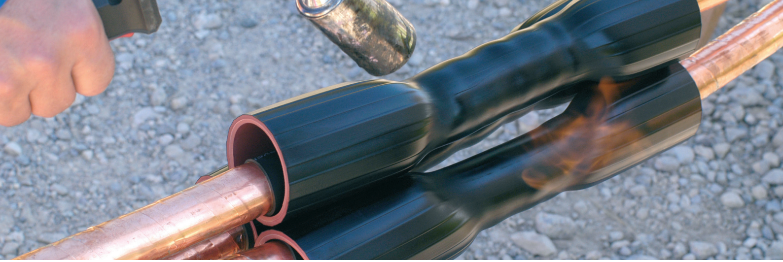
Rayfit tube used in MV Splices - Combines 3 layered, thick-wall extrusion.
